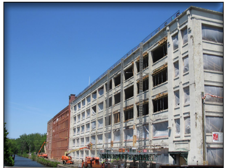
Ongoing construction at the Montgomery Mill TOD site.
