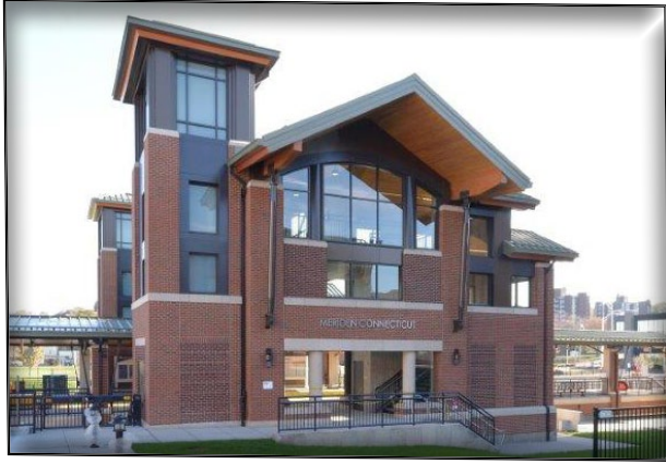
New station in Meriden.
