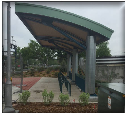
New bicycle racks at State Street Station.
