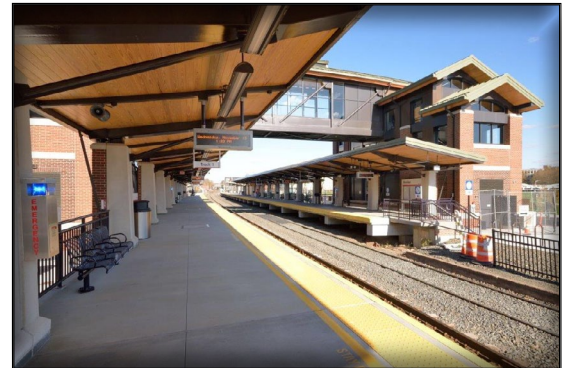
High-level platform at the new Meriden Station.
